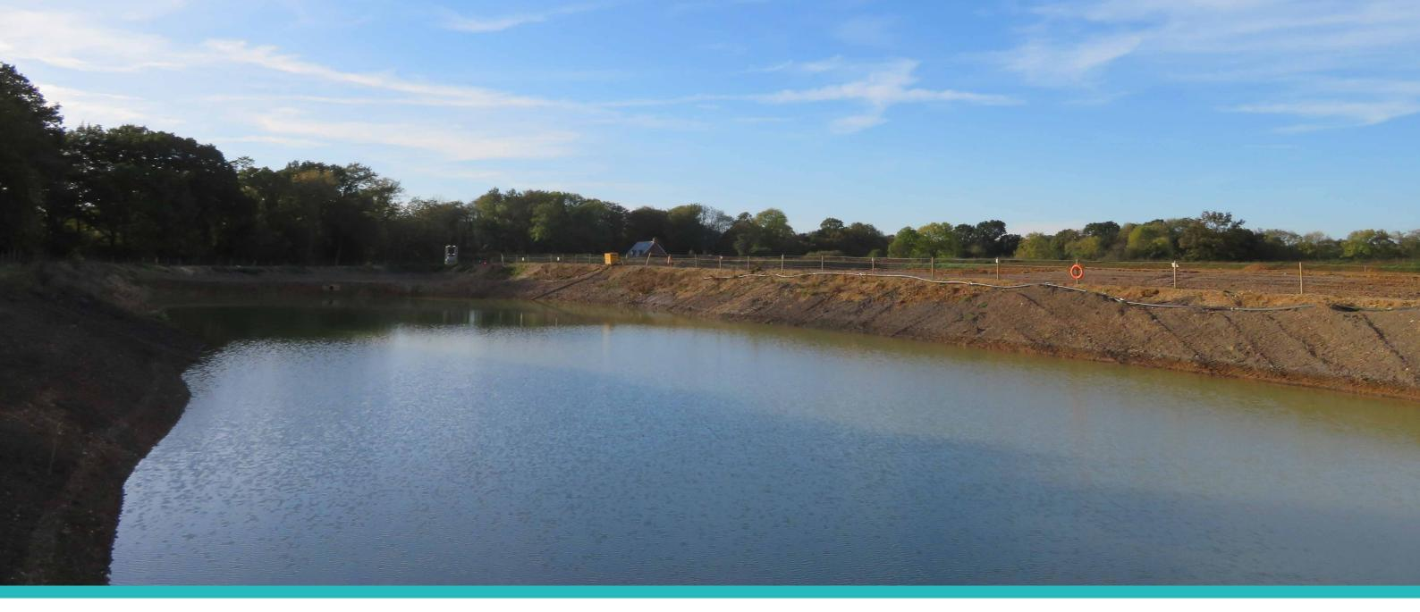
Upgrades to Roke Manor Quarry as Tipping commences in Phases 2 and 3 The newly constructed Phases 2 and 3 of the quarry have now been lined with clay and are receiving inert construction arisings. It is intended that the cells will be filled and the topsoil laid in the new year, with the first crop of grass sown in spring. As the site enters a very busy period of tipping, a number of other improvements have also been made to the site to accommodate this.
